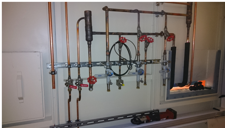
Figure 8: The inside wall of the hutch facing the storage ring. The figure shows the incoming pipes for the gas system from the cabinets outside. To the right, a chicane without its cover is shown.
