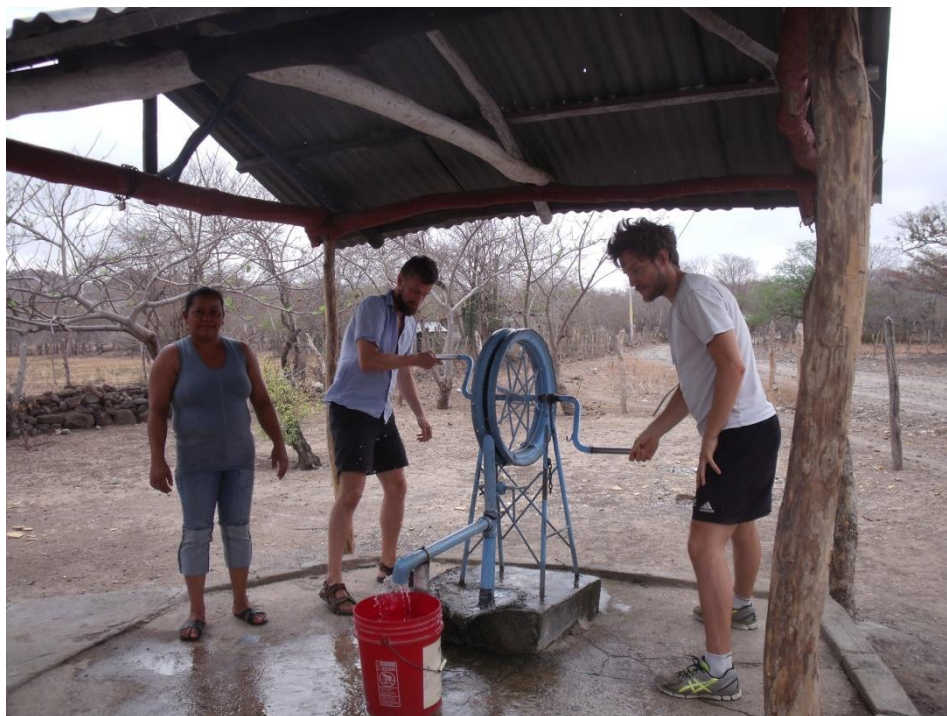
Figure 17 Typical hand pumped well in the village El Llanito.
