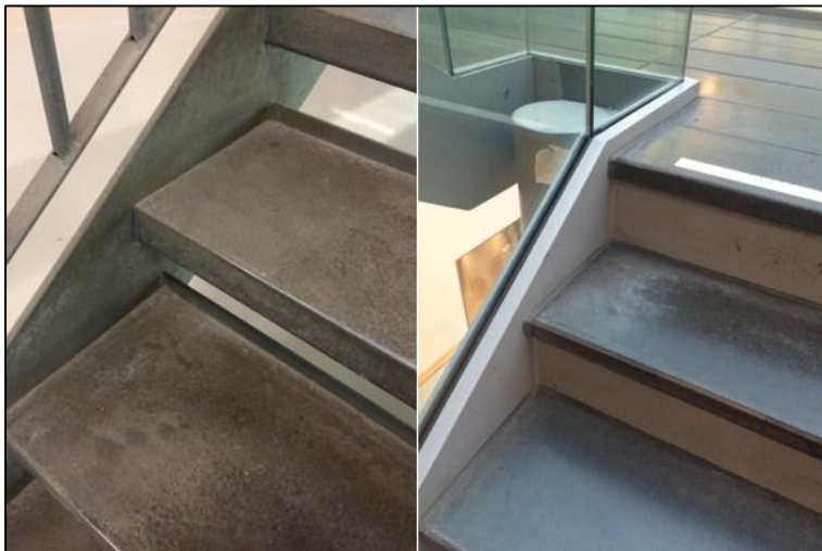
Figure 6.11. Treads with infill at Ubåtshallen and Malmö Höghskola Orkanen in Malmö.
