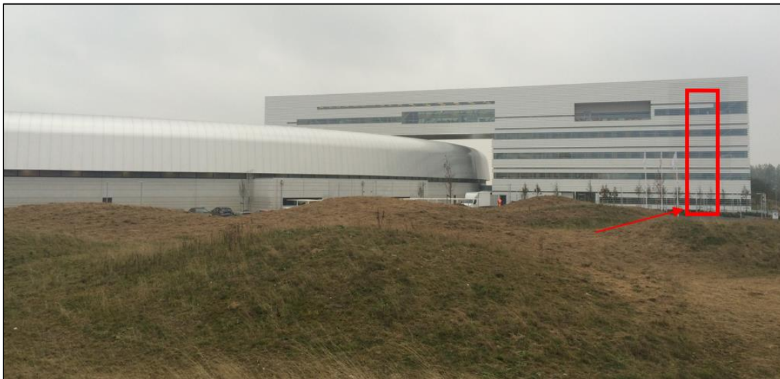
Figure 3.1. Position of the staircase(marked with red box) with marking(arrow) of test floor.
