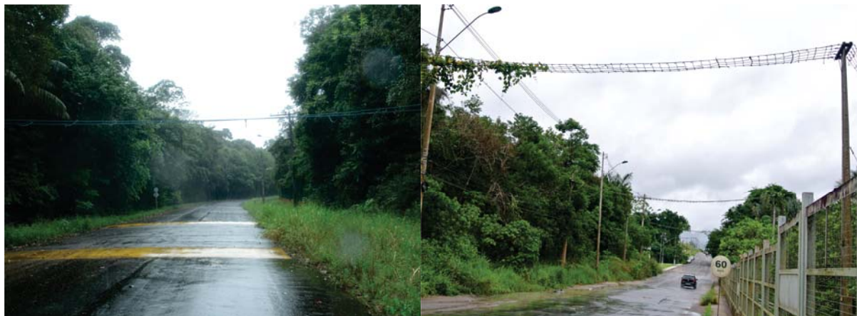
Fig. 14. Left photo displaying best solution for overpass, as seen in Ponta Negra. Good rope ladder, speed bumps around overpass and warning signs with reduced speed before and after. The picture is from the north-western part of Manaus, in a newly constructed settlement in Ponta Negra. On the right, the photo displays a good example of rope ladder. Designed like ladder, with many ladders next to one another. Vines will grow upon them for good camouflage and natural looking passage. Speed bumps exist and reduced speed with warning signs of wildlife crossing. Picture from industrial area outside central Manaus (Photos by S. Barr).
