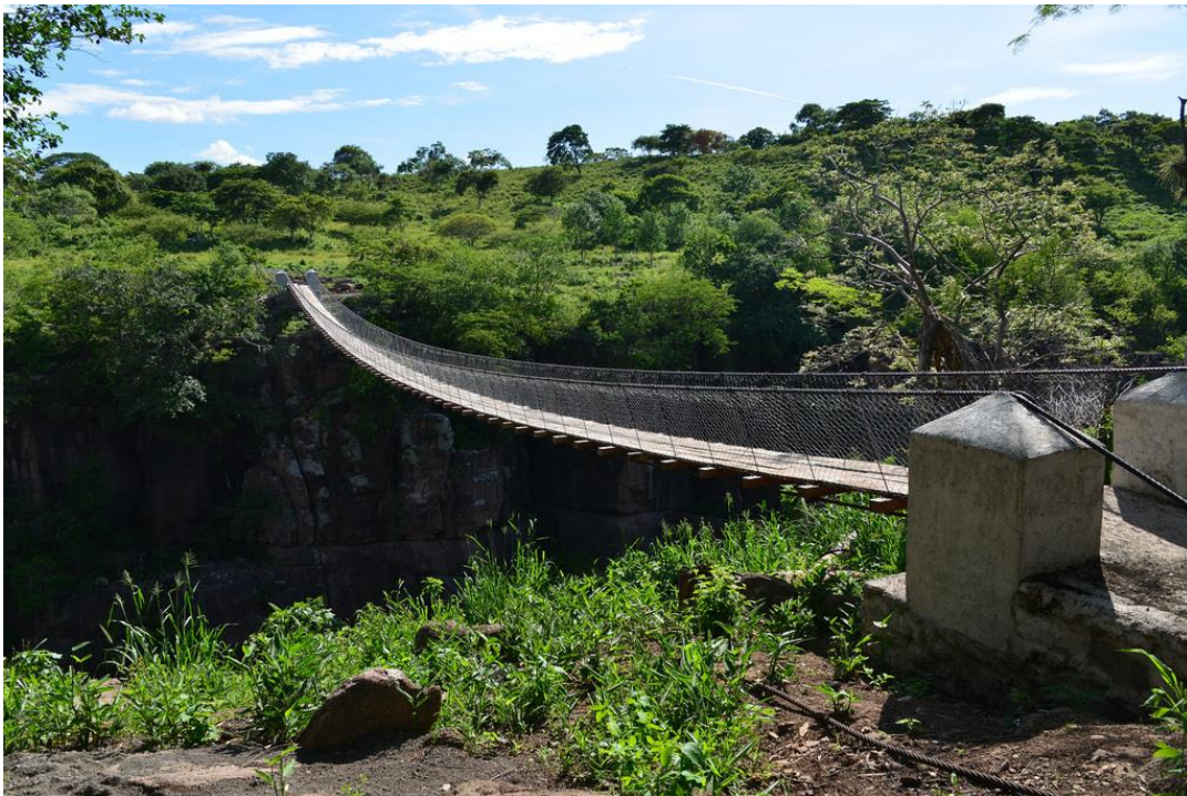
Figure 3.1 The Jicaro Bridge
