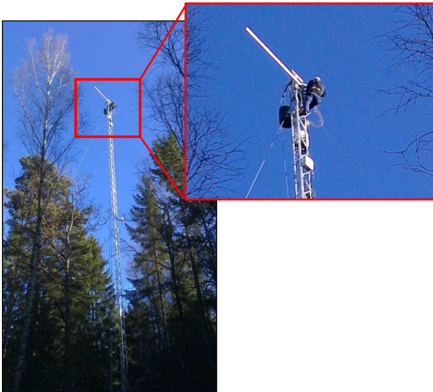
Figure 1. The Romperöd flux tower during maintenance.
