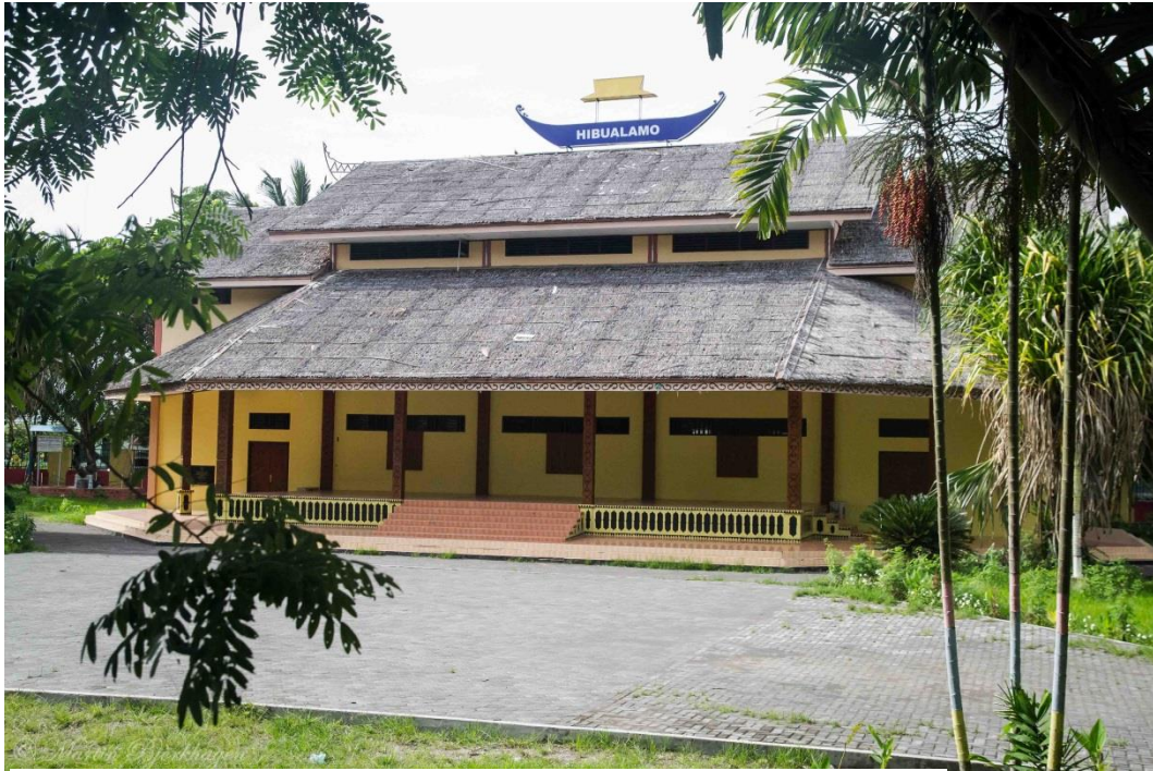
The newly-built Hibualamo in Tobelo City, finished in 2007, on the initiative of Hein Namotemo's regency administration, in NHR.
