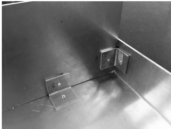
Figure 11.10 Corner pieces attached by pop rivets used for assembly
