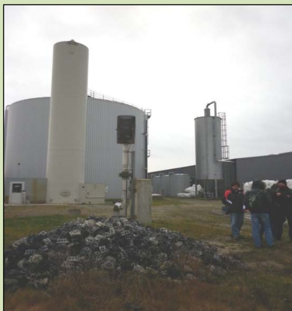
Scrubber and biogas reactors at Biokraft, Aakirkeby.
