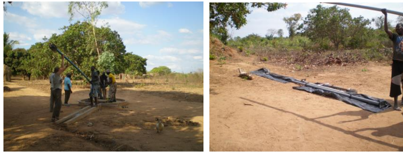
Figure 4-36 Dismounting of the pump tube at Naholoco EP1-2 (left) and Camaculo (right).
