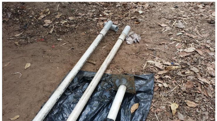
Figure 29 Riser pipes laid out on plastics on the ground – exposed to outer contamination. Photo by Elin Olsson.
