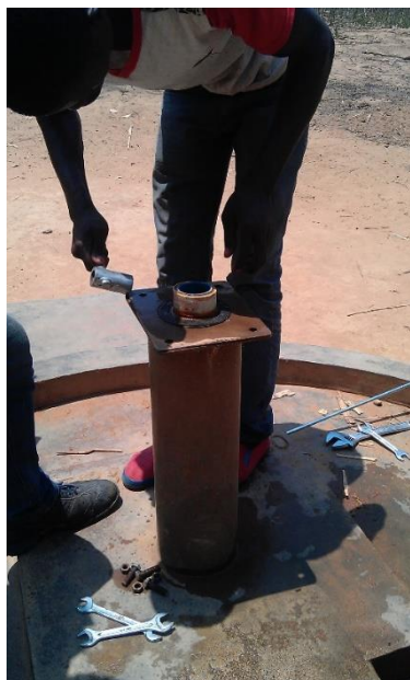
Figure 31 Top flange and above ground outer casing of the borehole. Photo by Elin Olsson.
