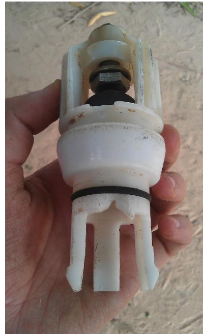
Figure 32 Broken footvalve – need for replacement. Photo by Elin Olsson.
