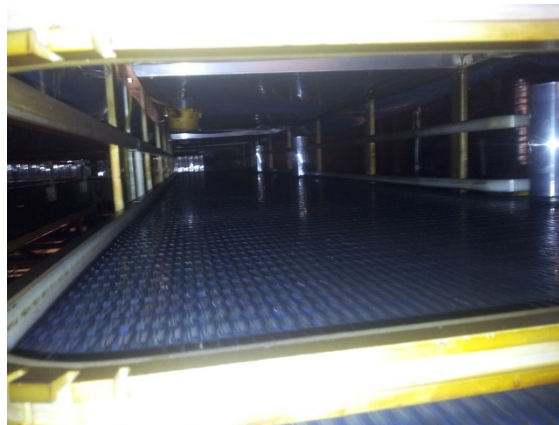
Figure 1.5. Empty conveyor belt.
