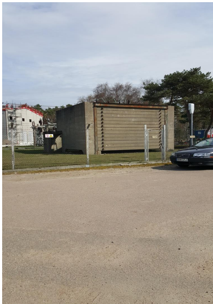
Figure 6. Example of sensitive parts being protected by a concrete casing.
