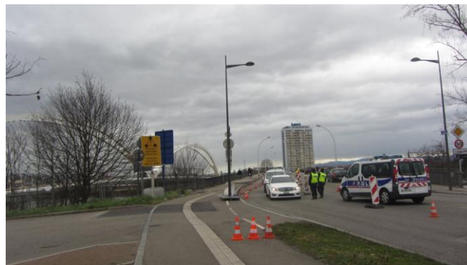
The new bridge for trams under construction on the left, pedestrians and cars crossing le Pont de l'Europe , the French-German border, Strasbourg, France. (2016, February 8).
