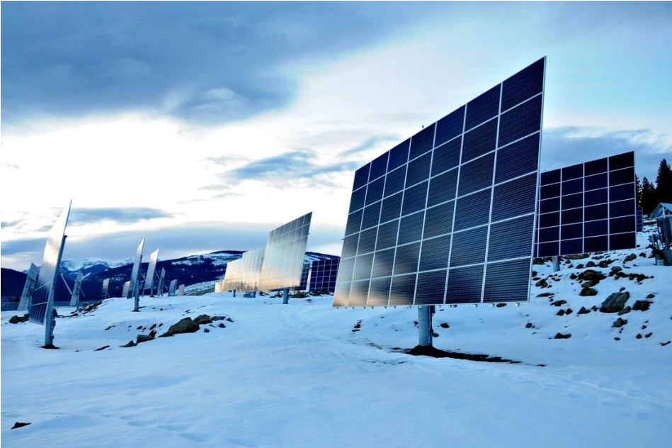
SunMine in the winter. Panels are tilted fully forward to catch the last of the day’s light (City of Kimberley, 2016).
