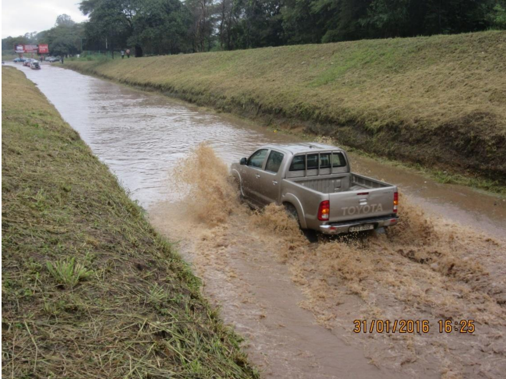
Figure 3: Southern side of Underbridge on Dag Hammarskjöld Drive
