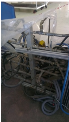
Figure 11. Old leak test manifold.
