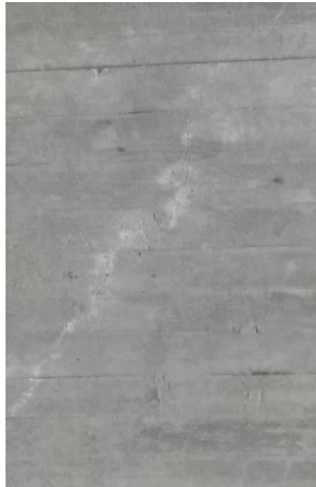
Figure 92 - Cracks in bridge 12-598-1. Left is front wall and right is valve.
