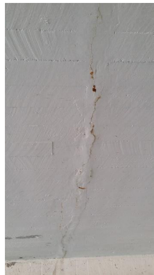
Figure 95 - Cracks in bridge 12-606-1. Left is front wall and right is valve.
