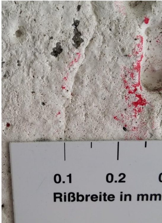
Figure 96 - Cracks in bridge 12-650-1. Left is front wall and right is valve.
