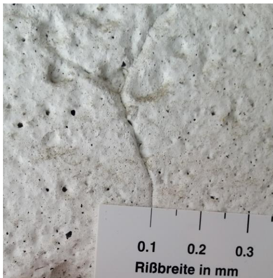
Figure 95 - Cracks in bridge 12-606-1. Left is front wall and right is valve.
