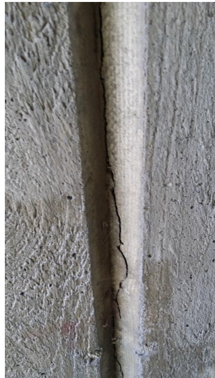
Figure 97- Cracks in bridge 12-921-1. Left is front wall and right is construction joint for front wall.
