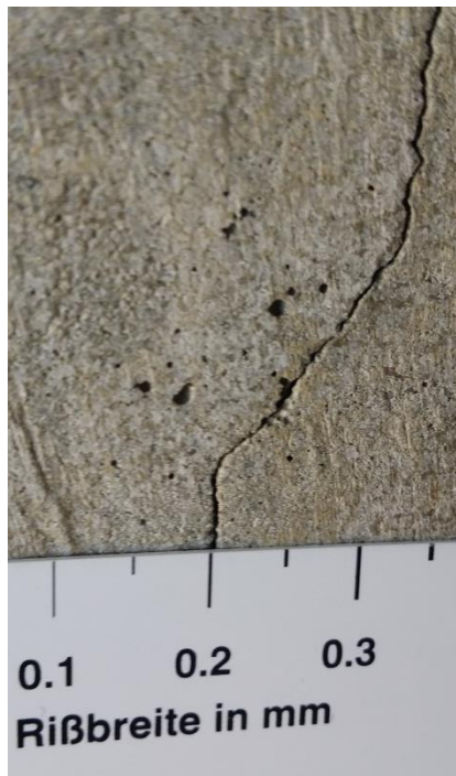
Figure 92 - Cracks in bridge 12-598-1. Left is front wall and right is valve.
