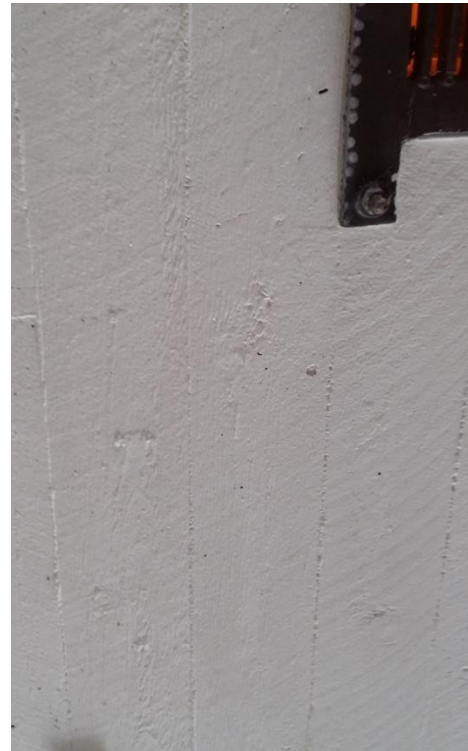
Figure 96 - Cracks in bridge 12-650-1. Left is front wall and right is valve.
