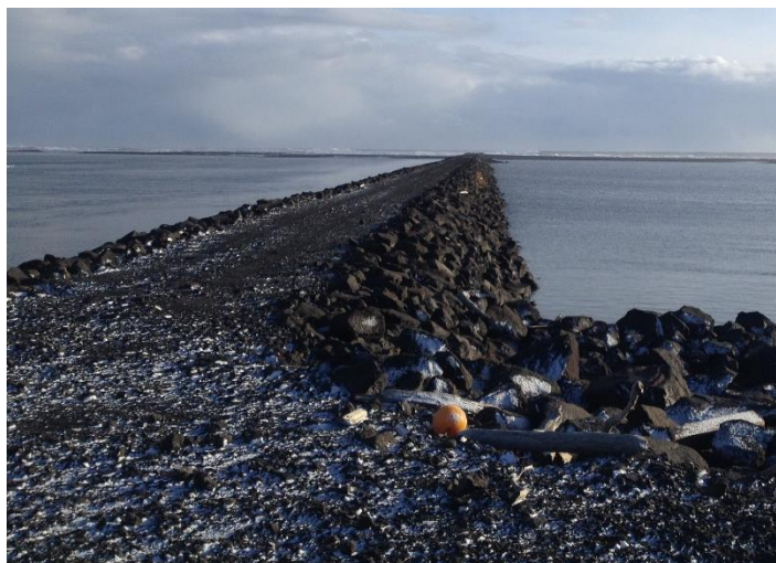
Figure 6: The wall constructed close to the harbour to divert the outlet of the river Markarfljót to a more eastern location.
