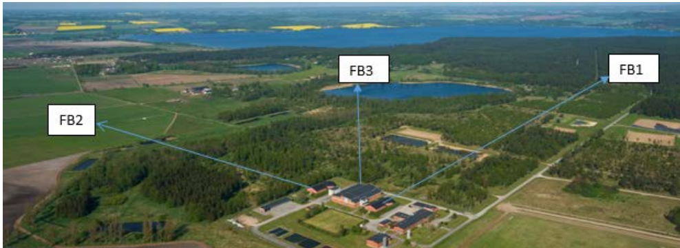
Figure 5-1: Vombverket aerial view
