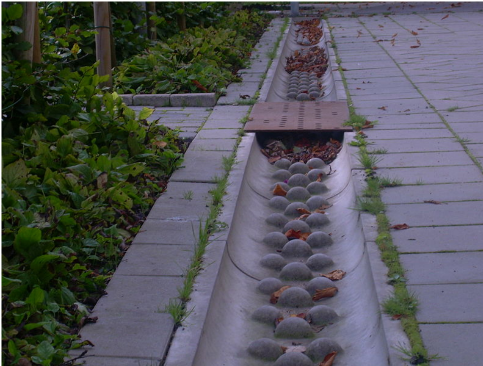
Figure 4-3 An empty drainage canal in Augustenborg
