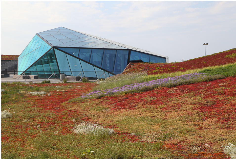
Figure 4-10 Roof park on Emporia Shopping Center, Hyllie
