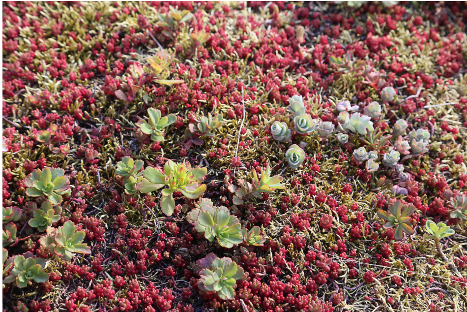
Figure 4-11 Sedum mat on Emporia green roof
