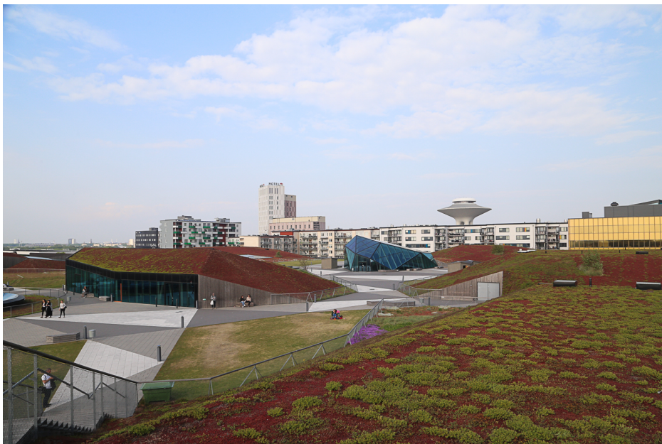
Figure 4-9 Roof park on Emporia Shopping Center, Hyllie
