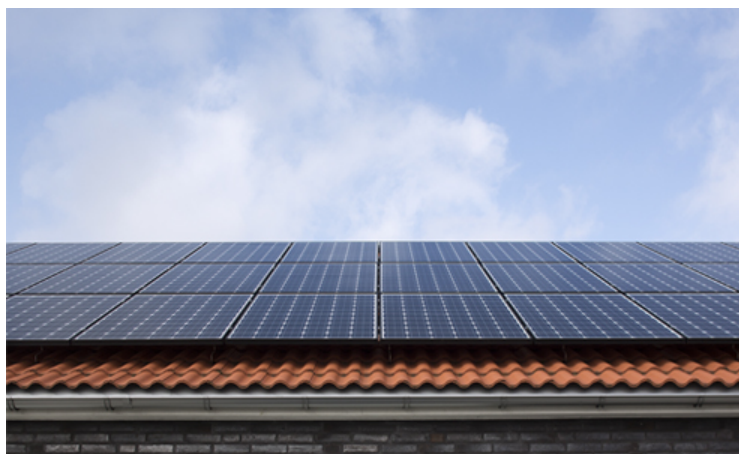
Figure 3.5: A large array of solar panels installed on a roof. Photo: Kraftringen [35]
