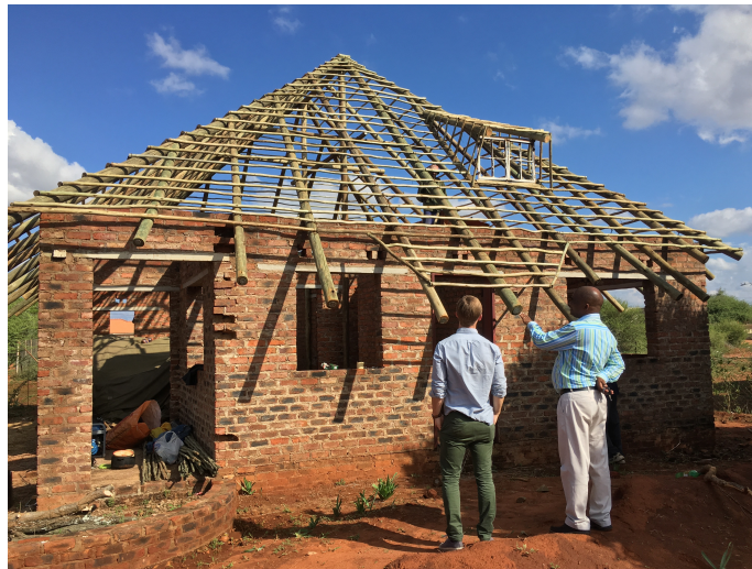
Figure 1.3: Inspection of a residential house under construction in Gaborone led by Dr. Rakgati.
