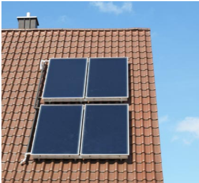
Figure 3.2: Typical installation of flat plate collectors on a roof. Photo: SolarShop [31]
