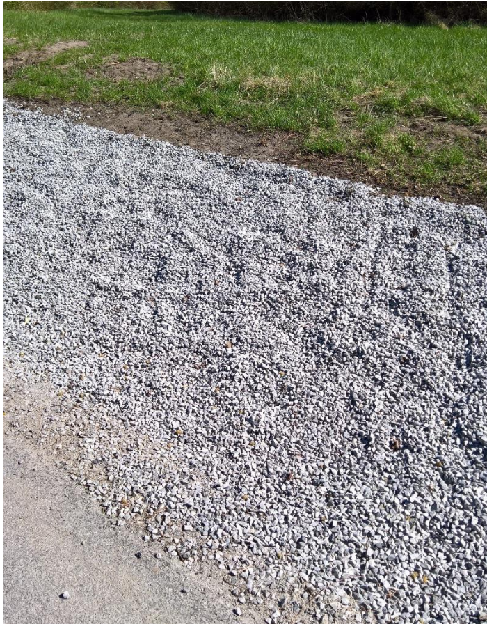
Figure 49 small gravel test
