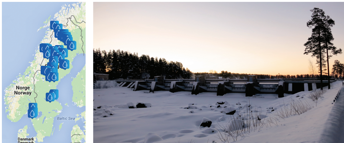
Figure 1.1: Left: Vattenfall's hydro power plants in Sweden [26]. Right: Hydro power plant in Älvkarleby during winter (Photo: Martin Rosenqvist)
