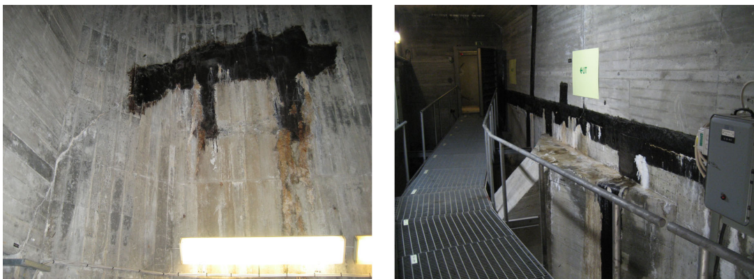
Figure 2.6: Repaired cracks in hydro power stations (Photo: Martin Rosenqvist)
