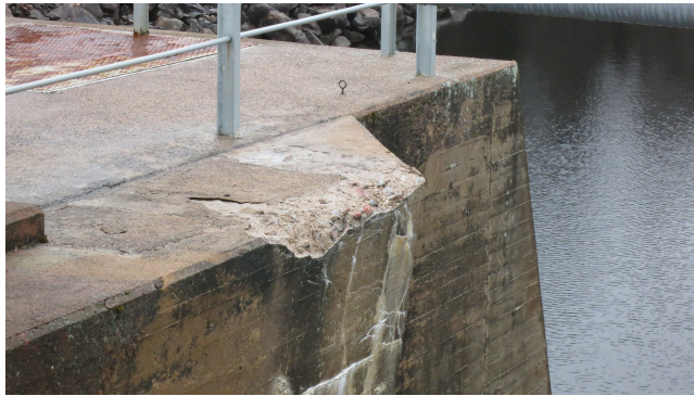
Figure 2.7: Internal frost damage causing a corner in a hydro power station to fail (Photo: Martin Rosenqvist)
