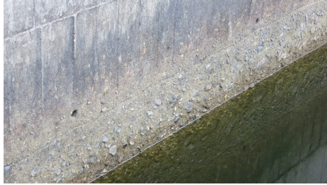
Figure 2.8: Example of surface scaling at the waterline (Photo: Martin Rosenqvist).
