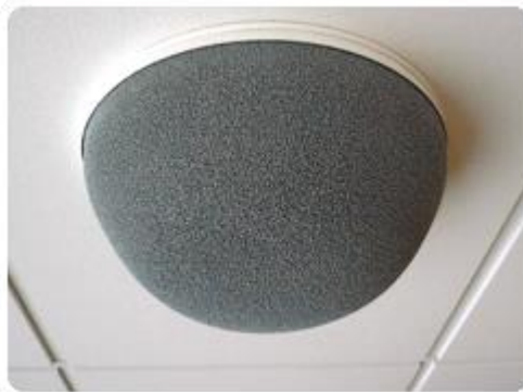
Figure 11 – Airson Airshower displacement ventilation diffuser
