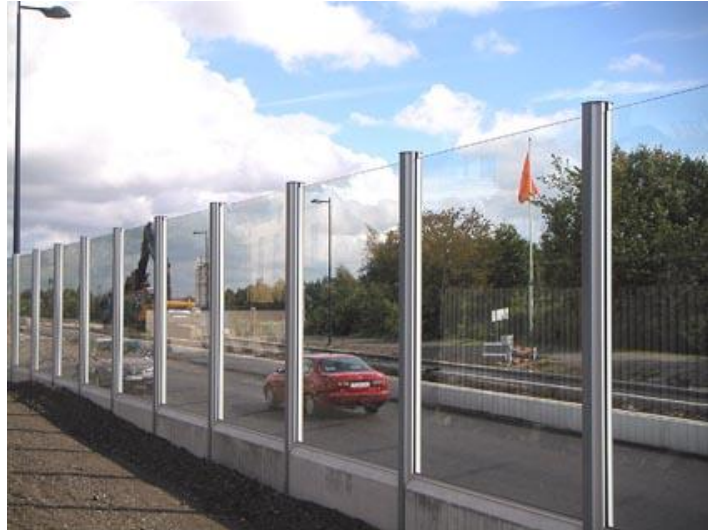
FIGURE 10. NOISE BARRIER ALONG BUSY ROAD (BULLERSKÄRM, 2014).
