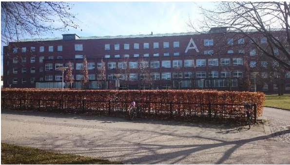
Figure 5: A-building (Photo by the author)
