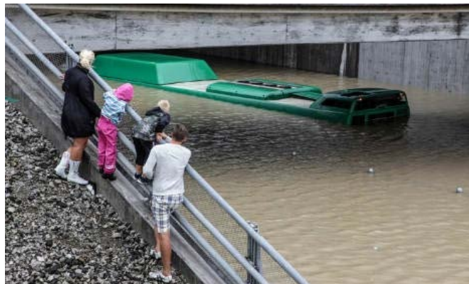
Figure 1-1 Malmö was flooded by a cloudburst event in August 2014
