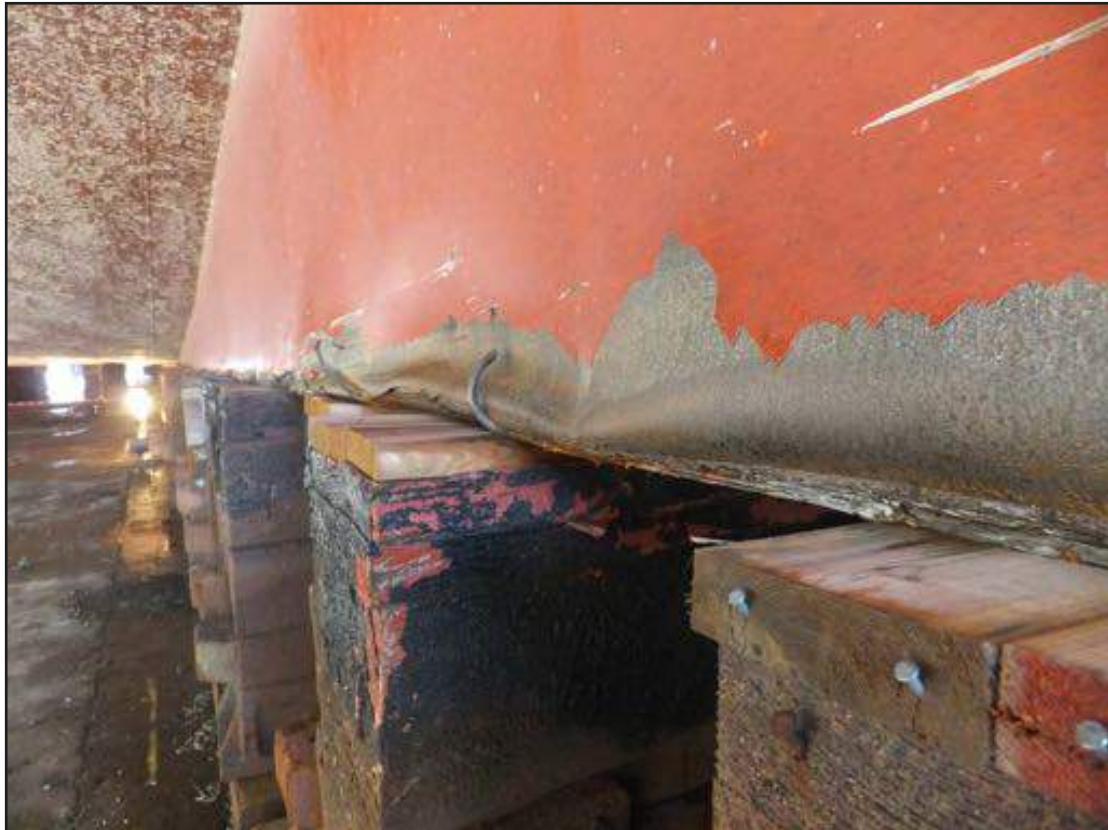
Figure 11: Detail of damage to keel skeg
