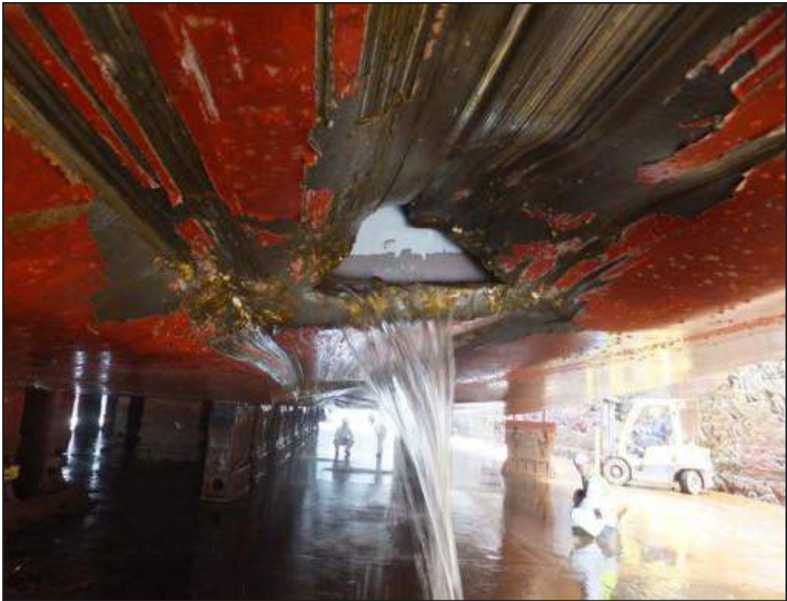
Figure 9: Second hole in water ballast tank 4
