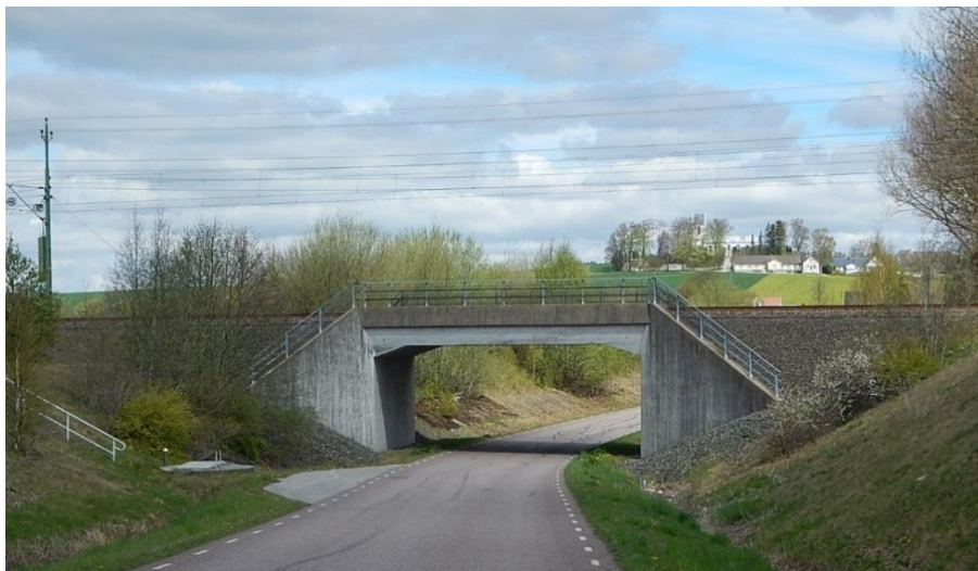
Figure 1.2: Portal frame bridge in Dagstorp north of Lund. From BaTMan (2015).
