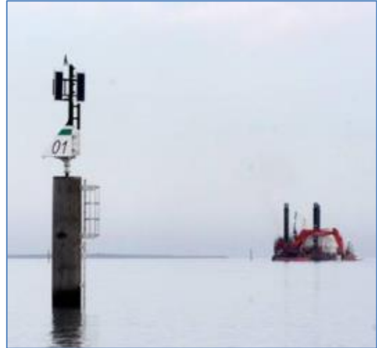
Figure 1: Dredging and placing HIB (Photo by: Olav Helge Matvik/Kystverket).
