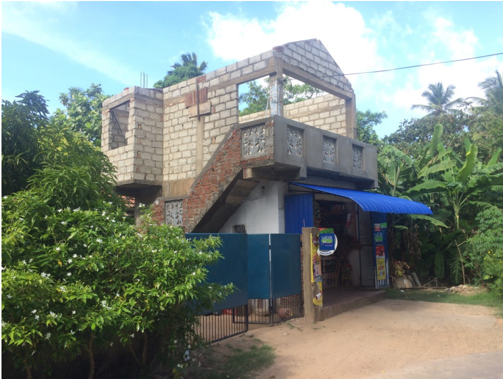
Figure B 1 – A building with a second storey used as shelter during floods.
