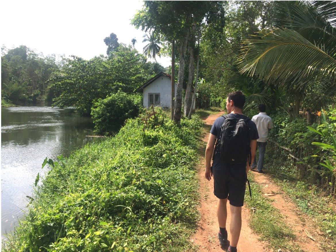
Figure B 3 - A picture from the research area with a flood prone house located right next to the river.
