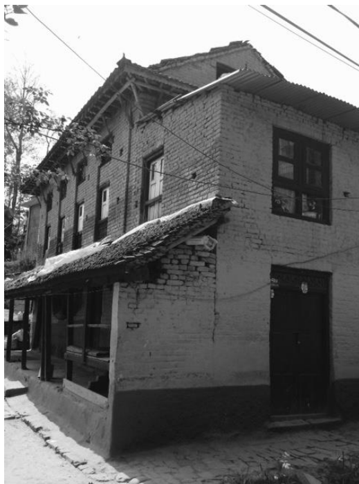
Figure 4.1: A traditional house in Dhulikhel made of dried bricks
