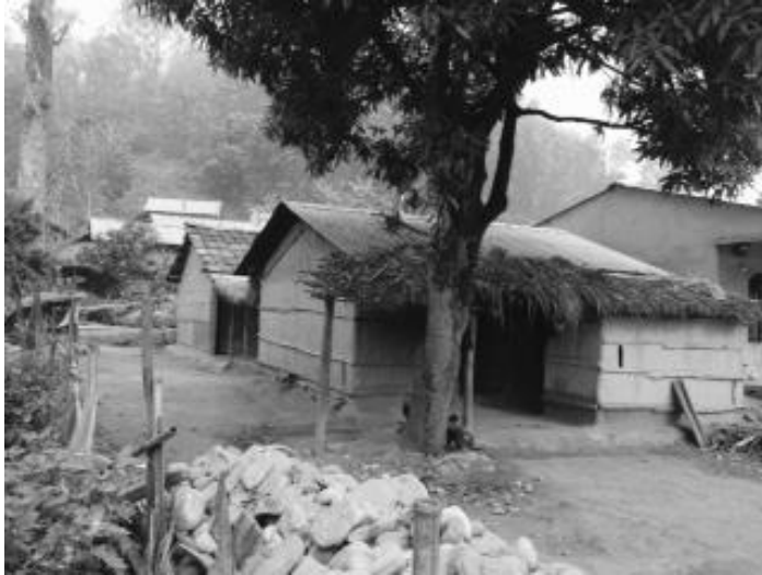
Figure 4.2: A traditional Taru house in Chitwan made of sticks and clay
