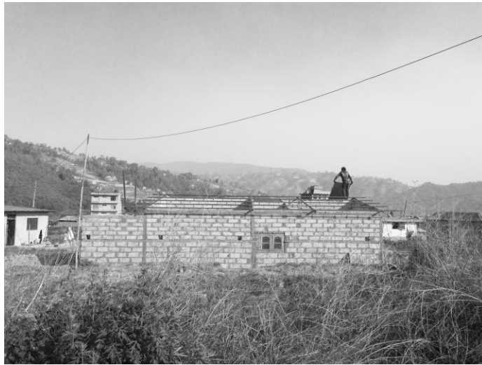
Figure 4.5: A house of concrete blocks under construction outside Pokhara
