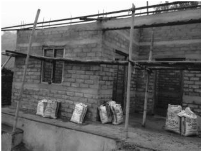
Figur 4.6: A house of compressed earth blocks under construction in Maji Gaun
