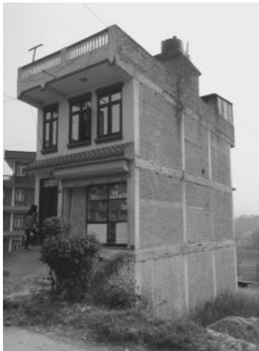
Figure 4.4: A reinforced brunt brick house in Dhulikhel
