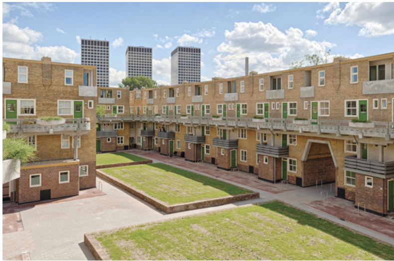
Bild 26, Spangen Rotterdam (architectural record 2014)
