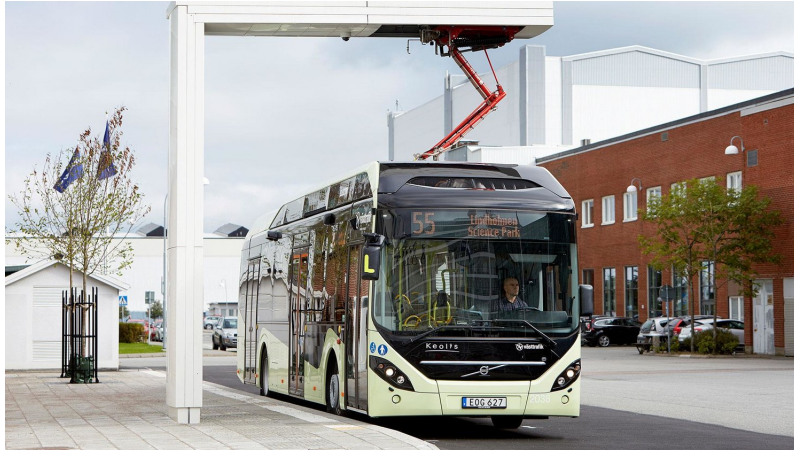
Figure 1: The L7900 electric bus being charged via the pantograph. [6]
