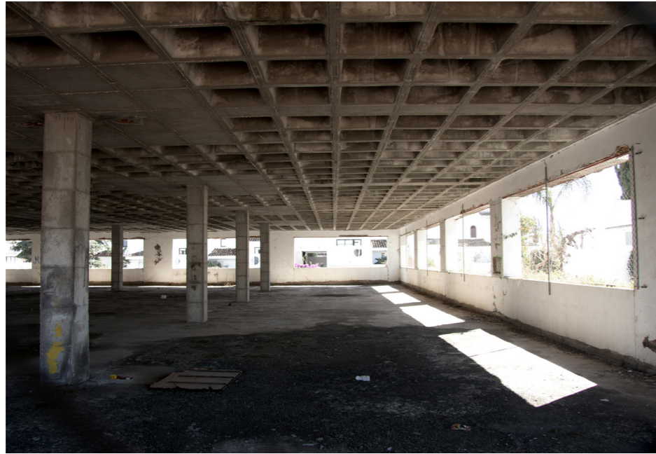
Photograph taken by author: Ground floor of existing building
