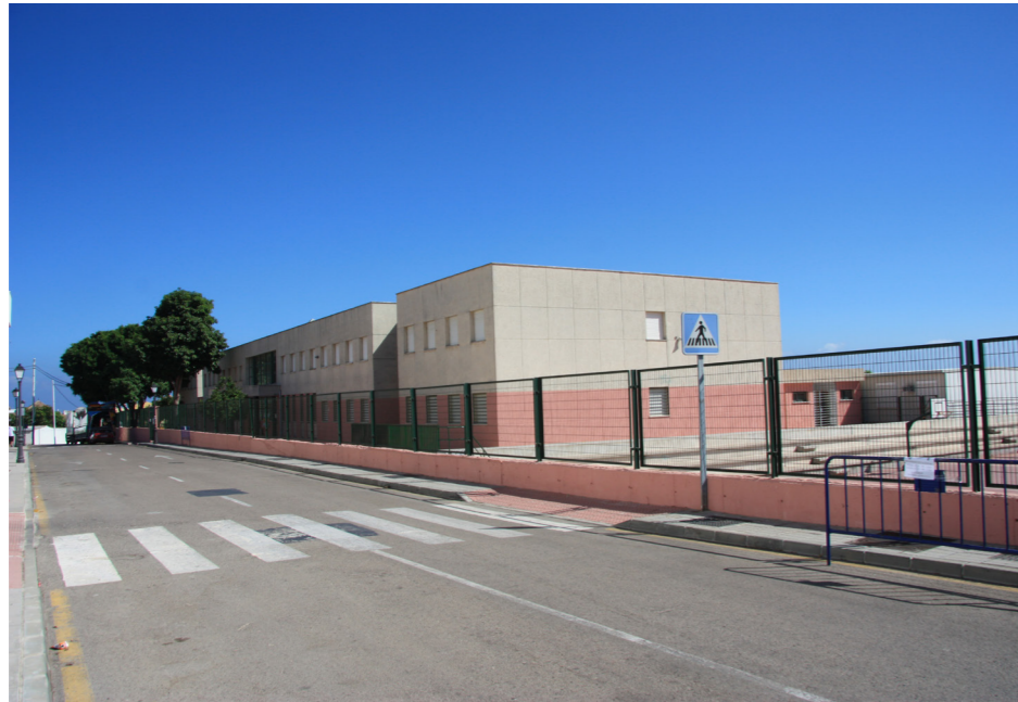
Photograph taken by author: Cancelada Primary School
