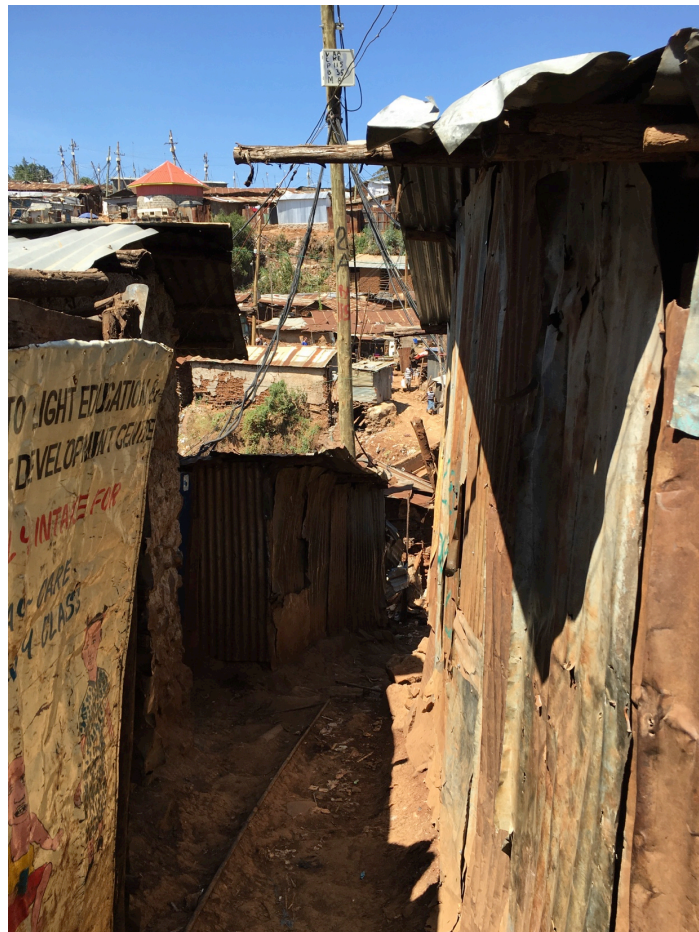
Figure 17: Inadequate infrastructure and poor housing (authors picture)
