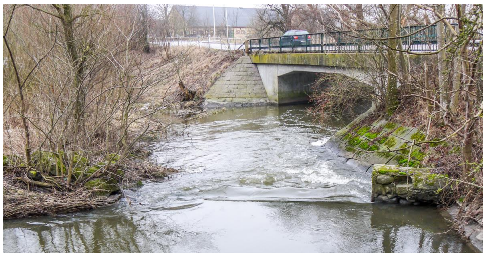
Figure 6.2: Trolleberg weir. Photo taken 31st of January 2017
