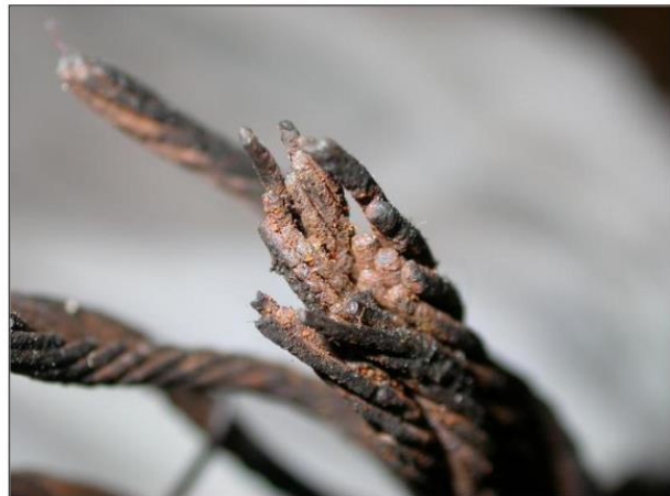
Figure 24 shows a close up of the internal corrosion on the wires, holding the lifeboat. Picture taken from: (Marine Safety Investigation Unit, 2014)
