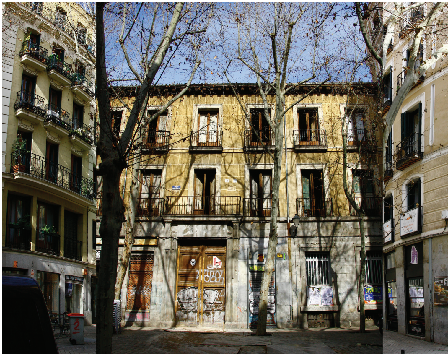
Main façade of the Palace of Sueca
