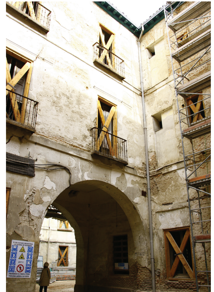
Access from first courtyard to second courtyard
