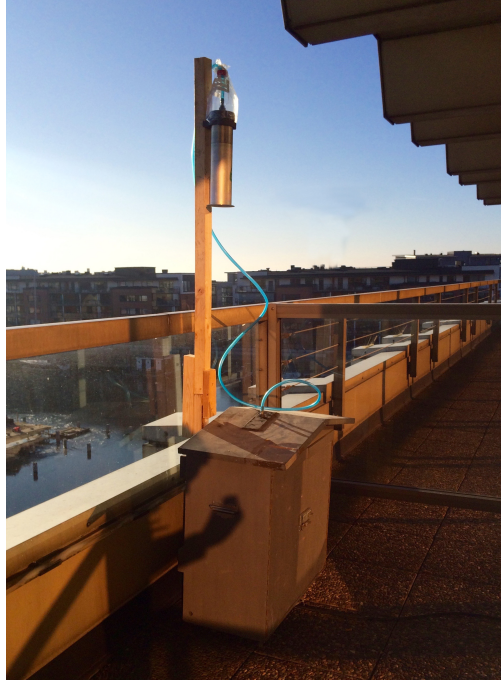
Figure 6: An image of the measurement setup located at Stadshuset.
