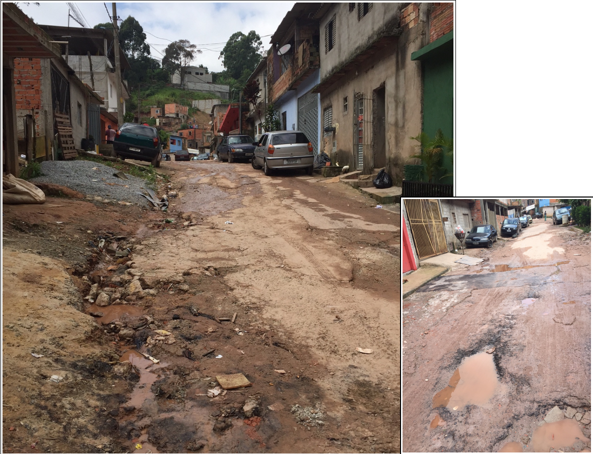
Figure 10. Photo of unpaved muddy street observed during field visit
