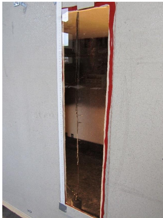
Figure 28: Window in test room.
