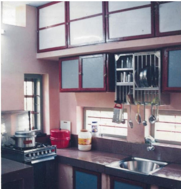
Left: The kitchen used recycled ventilators (openings above doors in a dismantled traditional house found at scrap shop) kept horizontally to give maximum natural light and ventilation for the working platform, with a view to pool. This is passively cooled and lit the kitchen throughout the day. Right: Wherever possible, wood and steel furniture was minimised using built-in brick furniture.
