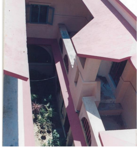
Left: dining hall arch with built-in brick diwan (rest platform by a pool) which cools the courtyard and house interior. Vent openings near ceiling above arch which allows warm air to escape as ventilation Right: rectangular courtyard in east-west direction. The rooms are built in north and south direction to minimise direct sunrays.
