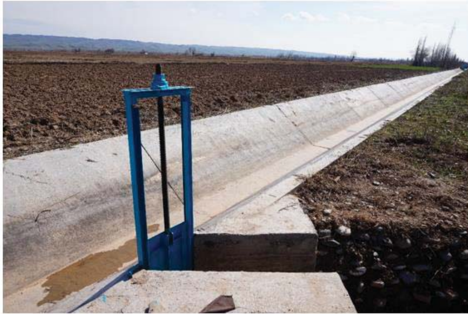
Figure 11. New irrigation channel and gates constructed using European funding in Alma-Suu WUA (03/17).
