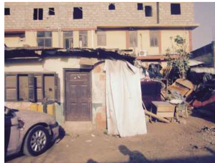
A badly deteriorated and abandoned building is sitting within the plot.
