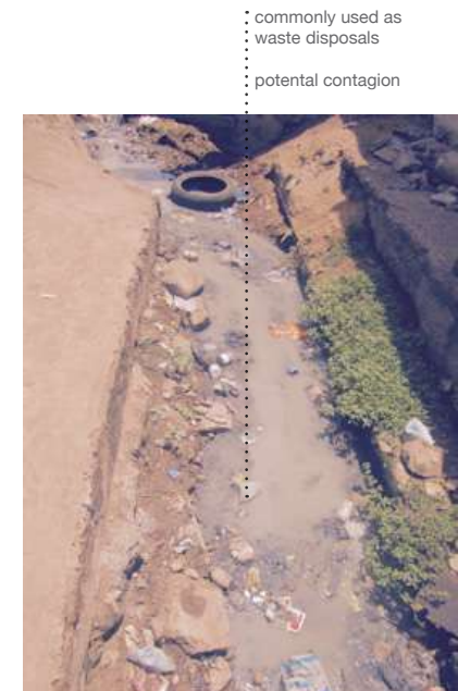
Nima's informal drainage system
