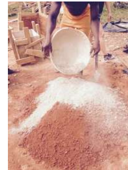
Soil mixed with cement, white sand and water.
