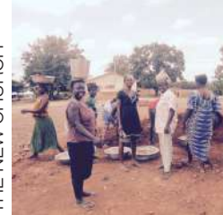
WOMEN BUILDING THE NEW CHURCH
