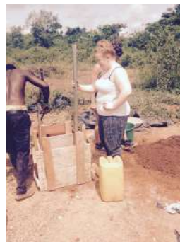
Earth is rammed inside formwork.
