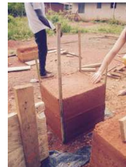
Formwork is removed. Finished Product.
