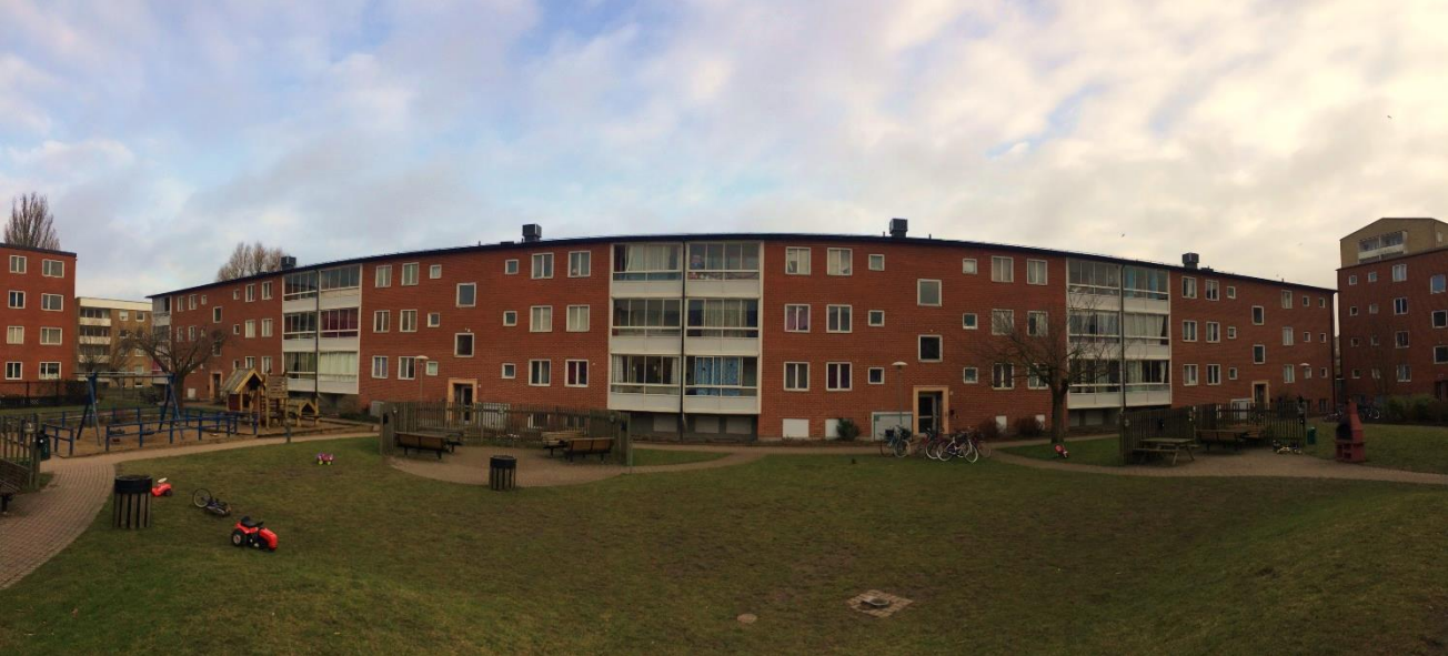
Figure 4.2. Panoramic view of the west side of the studied reference building.
