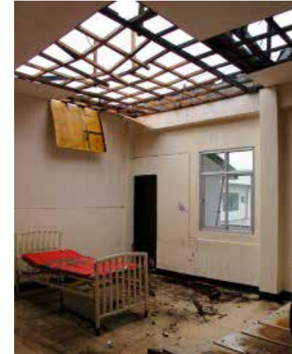
Fig 16: Ziga District Hospital in Tabaco destroyed by Typhoon Rammasun (Glenda) 2014 (Direct Relief, 2014)
