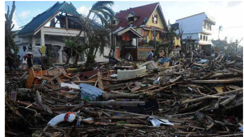
Fig 11: Destruction of the town Palo by Typhoon Haiyan 2013 (BBC, 2013)
