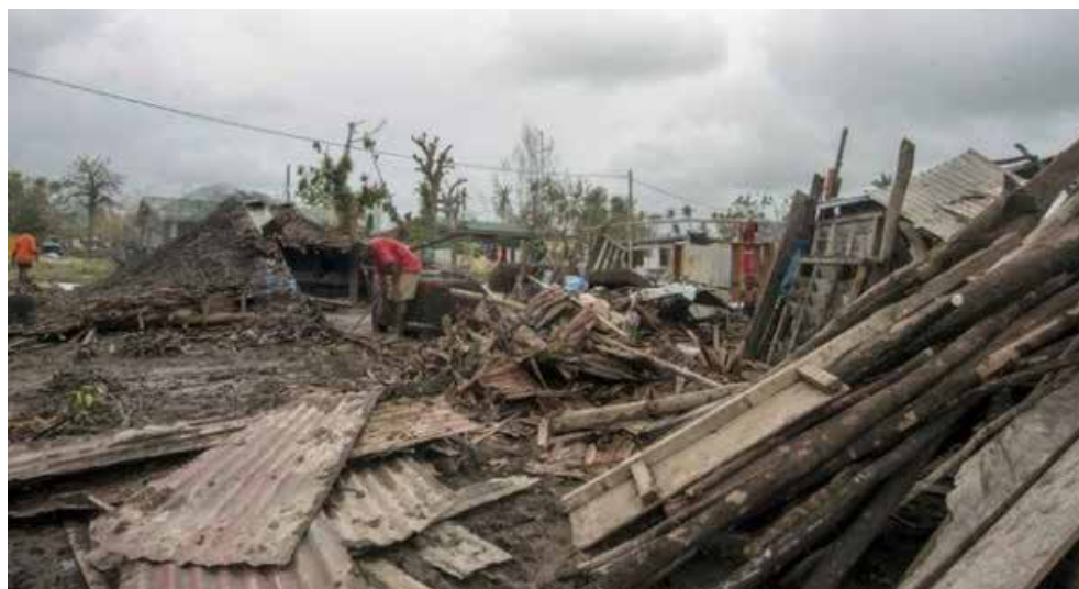
Fig 13. Destruction in Vanuatu by Cyclone Pam 2015 (newfrontierchronicle.org, 2015)
