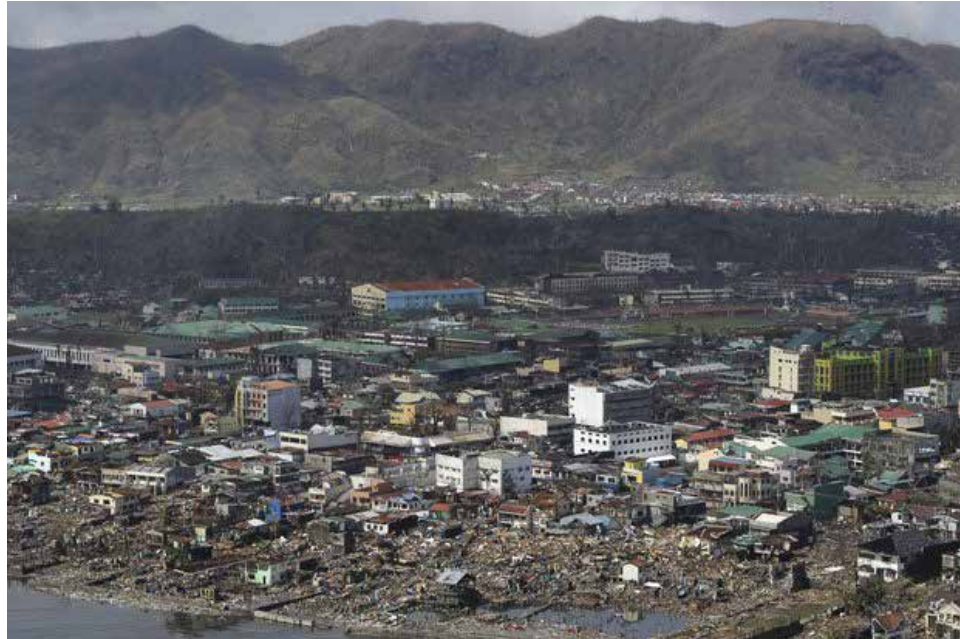
Fig. 37: Buildings that survived in Tacloban (globalnews.ca, 2013)
