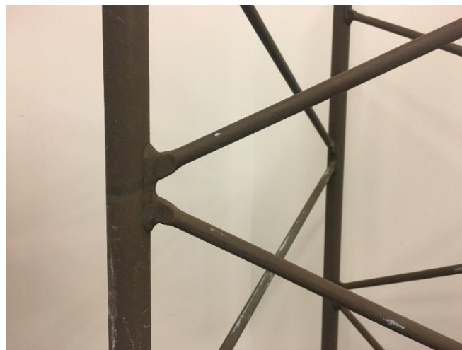
Figure 3.1 The truss found in Axis Installation Experience Center, is the same as the one found in many harbours. The poles are thicker than the webs.
