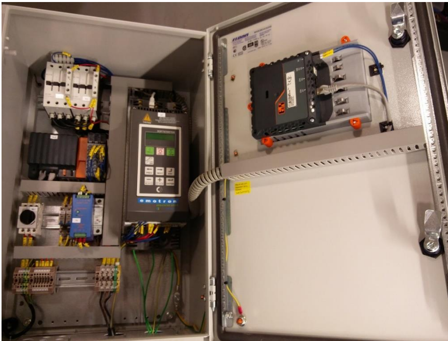
Figure 22. Open cabinet with all the components.
