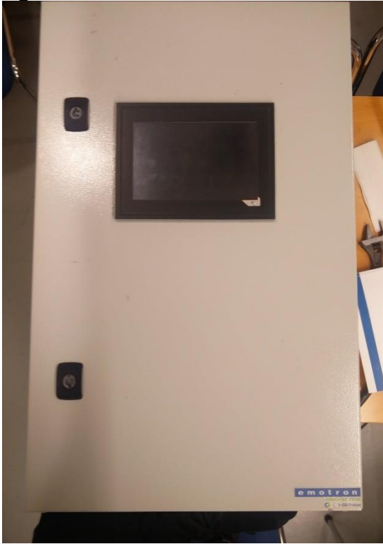
Figure 21. Closed cabinet from the outside.
